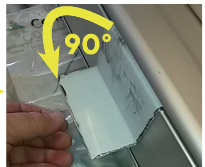
Rotate the bracket down
